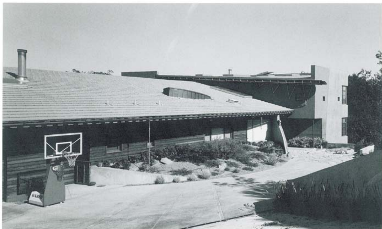
View toward entrance
