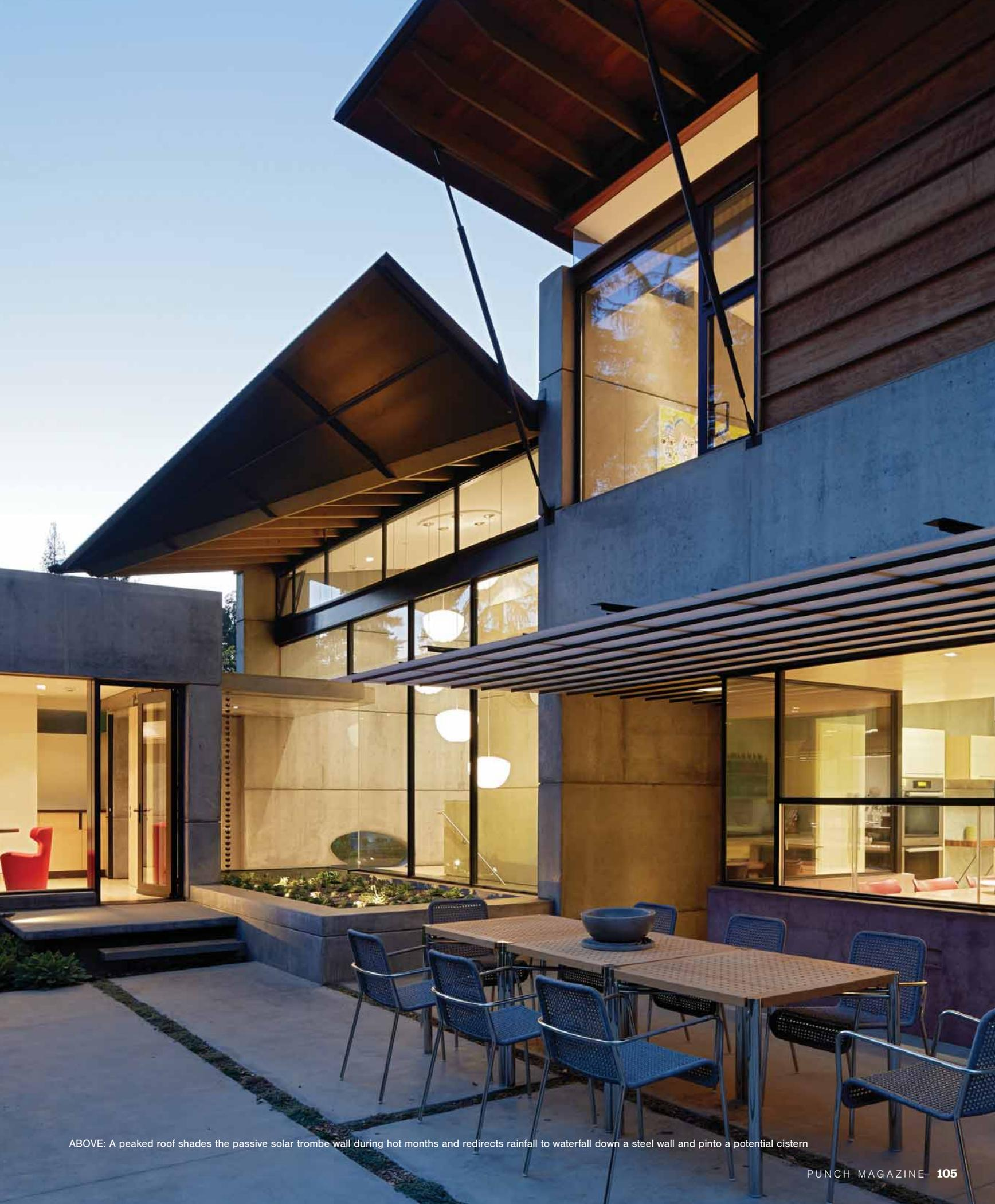
ABOVE: A peaked roof shades the passive solar trombe wall during hot months and redirects rainfall to waterfall down a steel wall and into a potential cistern
